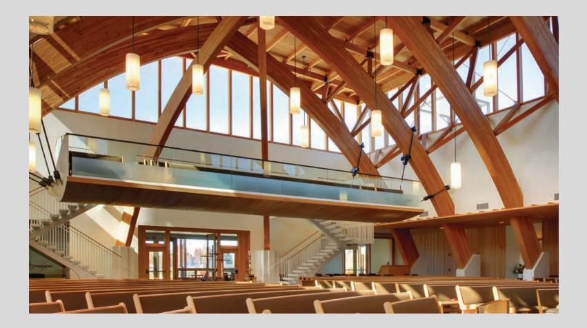
Glue laminated beams are made up of small pieces of wood, glued together, to form a composite, larger piece
